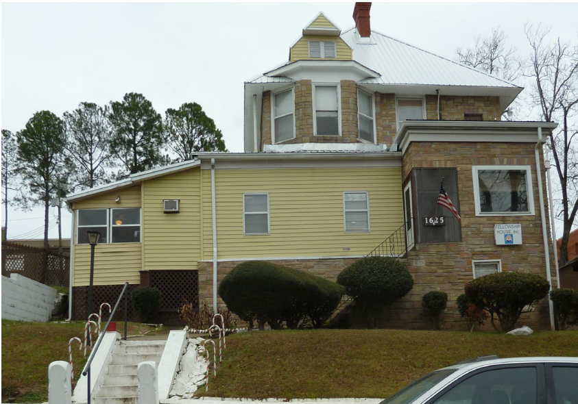
Example of an inappropriate addition to a historic structure (not in Anniston).
