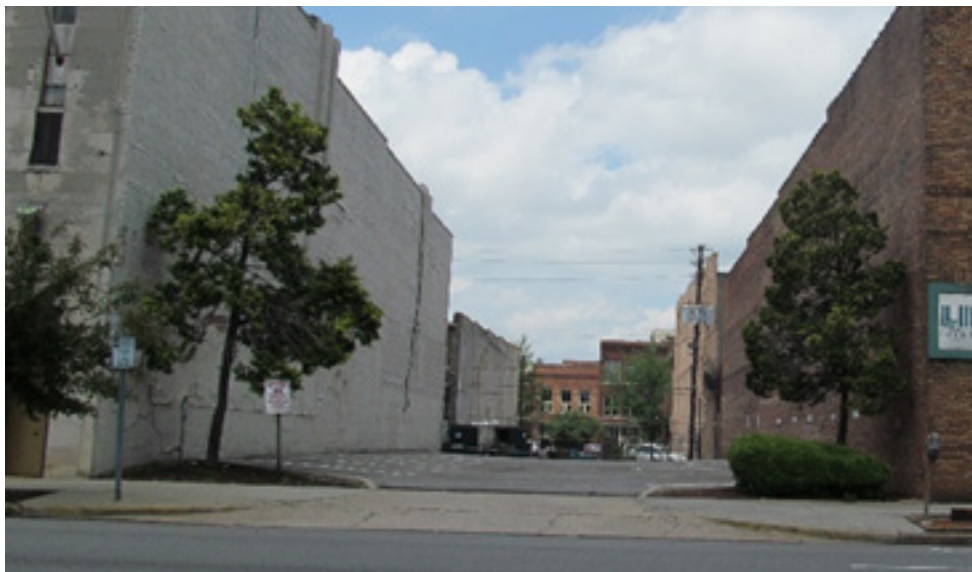
Example of how demolition can create inappropriate "snaggle-toothed" effect (not in Anniston).
