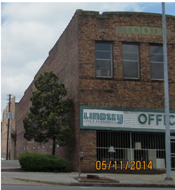
Many commercial buildings had built-in sign panels that should be repaired and retained. The plastic sign, however, is inappropriate and covers a historic transom window (not in Anniston).
