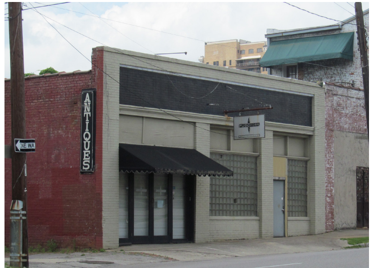
Example of inappropriate transom replacements (not in Anniston).
