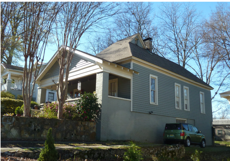
Example of a historic addition. This Queen Anne cottage has a ca. 1925 Craftsman porch that has historic significance even though it is not original to the home.
