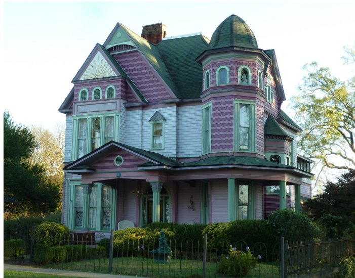
An excellent example of historic use of decorative wood siding and shingles.
