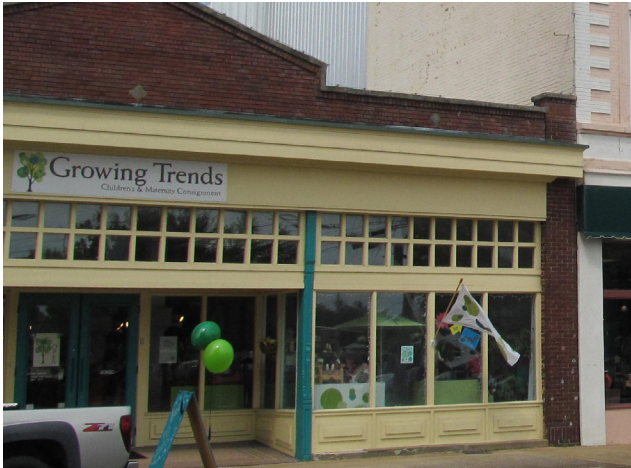
Example of typical Anniston storefronts with transoms.
