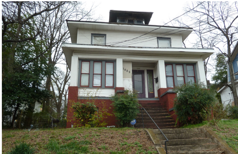
Example of an inappropriate porch enclosure (not in Anniston).
